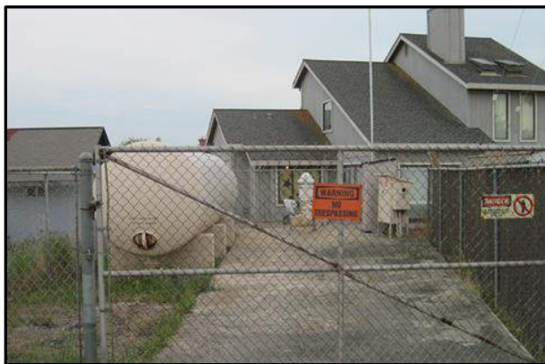
Figure 4.6 Photograph of Well 6
