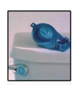
To determine if this is your problem, conduct a dye test using leak detection dye tablets or food coloring.
