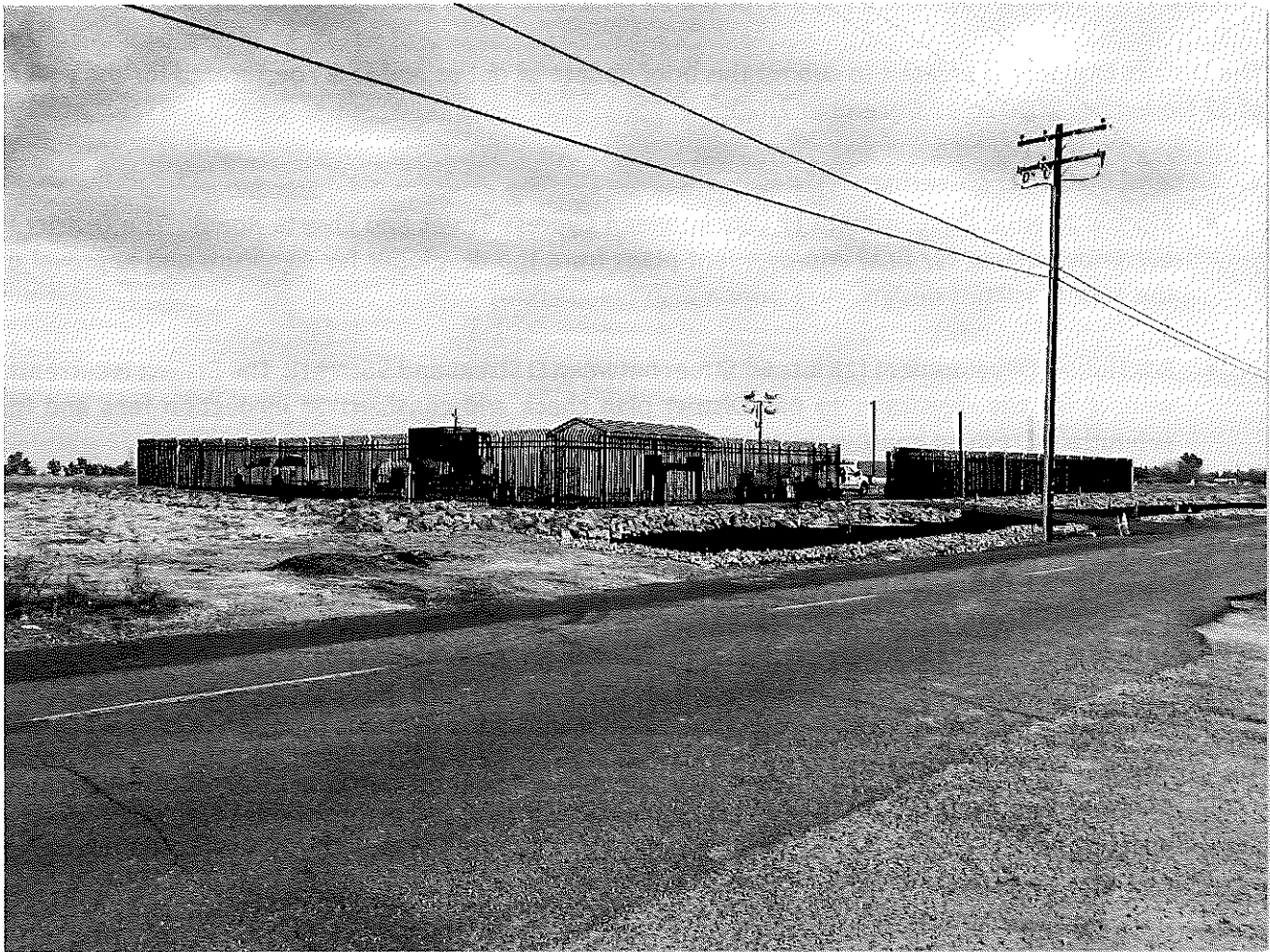
Well 16 site construction progress
